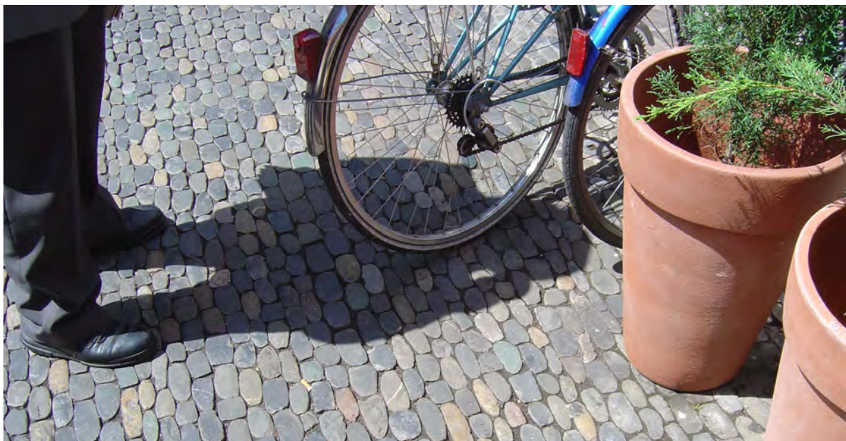
PERVIOUS COBBLE PAVERS, FREIBURG, GERMANY
