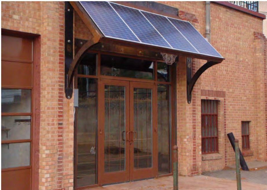
SOLAR COLLECTION SHADE STRUCTURE, DURANGO, CO
